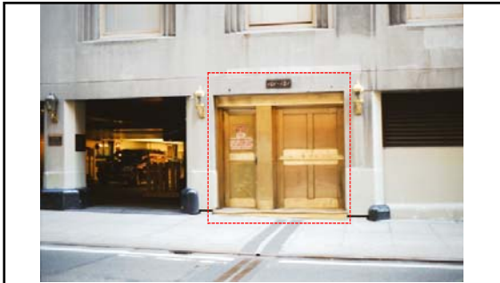
Elevator door (center) at 101-121 East 49th Street (2002). The matching bay/s to the left go to the hotel garage and the closed one (on the right) probably once did too (it has protective curbs). The elevator, by contrast, not only has no curbs but has a small, well worn step. 361
