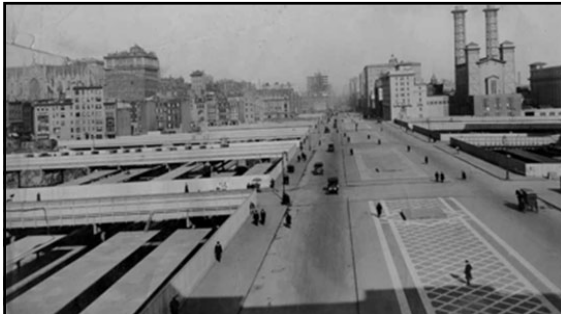
"While house wreckers are tearing down the old Grand Central Station the New York Central's staff of engineers and draughtsmen are finishing the plans which will extend Park Avenue northward from the new station to Fifty-seventh Street over what is now a deep gully threaded with the tracks of the new terminal system." The New York Times, June 26 th 1910 259
