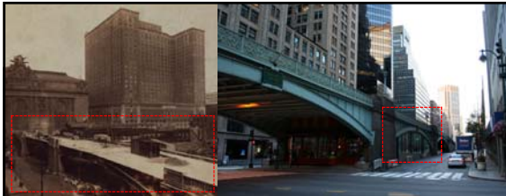
Left: Park Avenue Viaduct under construction in foreground (ca. 1918). Warren & Wetmore originally conceived the viaduct to have tall pylons; like that of the Alexander III Bridge (1900), but they were not realized. Right: each arch measures 200-feet in length for an overall length of 600-feet. The center arch (outlined) was enclosed at street level and presently houses a retail establishment (restaurant). 337
