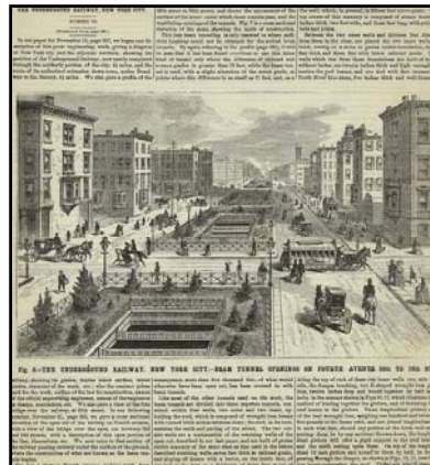
Left: newspaper article (ca. 1874) concerning the "Beam-Tunnel Operation on Fourth Avenue" (59 th to 76 th Street/s shown in drawing). It was more commonly referred to a "The Underground Railway."
