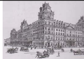
"...As a result of these complaints, in 1900 the station was enlarged to accommodate 60,000 passengers daily. The number of tracks was increased and three stories were added to the building. These changes cost over $2,500,000..."
