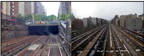
The 97 th Street tunnel portal, looking south - present-day (left). Between 97 th and 99 th Street/s, the tunnel emerges onto the Harlem viaduct (right) to the Park Avenue Lift Bridge which carries four tracks across the Harlem River into the Bronx and points north of New York City.
