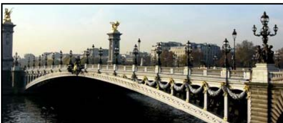
"Traffic will be carried over Forty-second Street at this level by a bridge, which will be an exact copy of the famous Alexander III Bridge over the river Seine in Paris. This structure, which was erected several years ago in honor of Alexander III of Russia, is said to be one of the most beautiful in the world."
